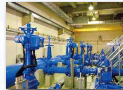
Sewage treatment plant
