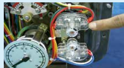
Limit switch inspection
