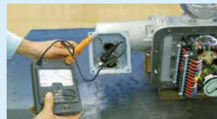
Electrical insulation measurement
